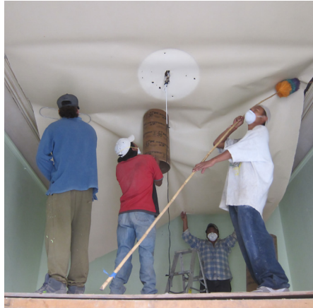
Plafond removal in Edison 169. July 4, 2013, 8:42 hrs.
