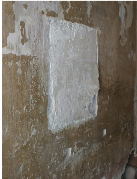
Removal process of a wall in Tonalá 47. April 8, 2006, 13:04hrs.
