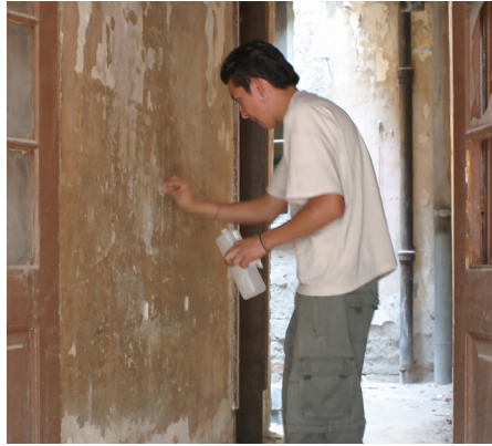
Removal process of a wall in Tonalá 47. April 7, 2006, 10:01hrs.
