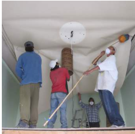
Plafond removal in Edison 169. July 4, 2013, 8:42 hrs.
